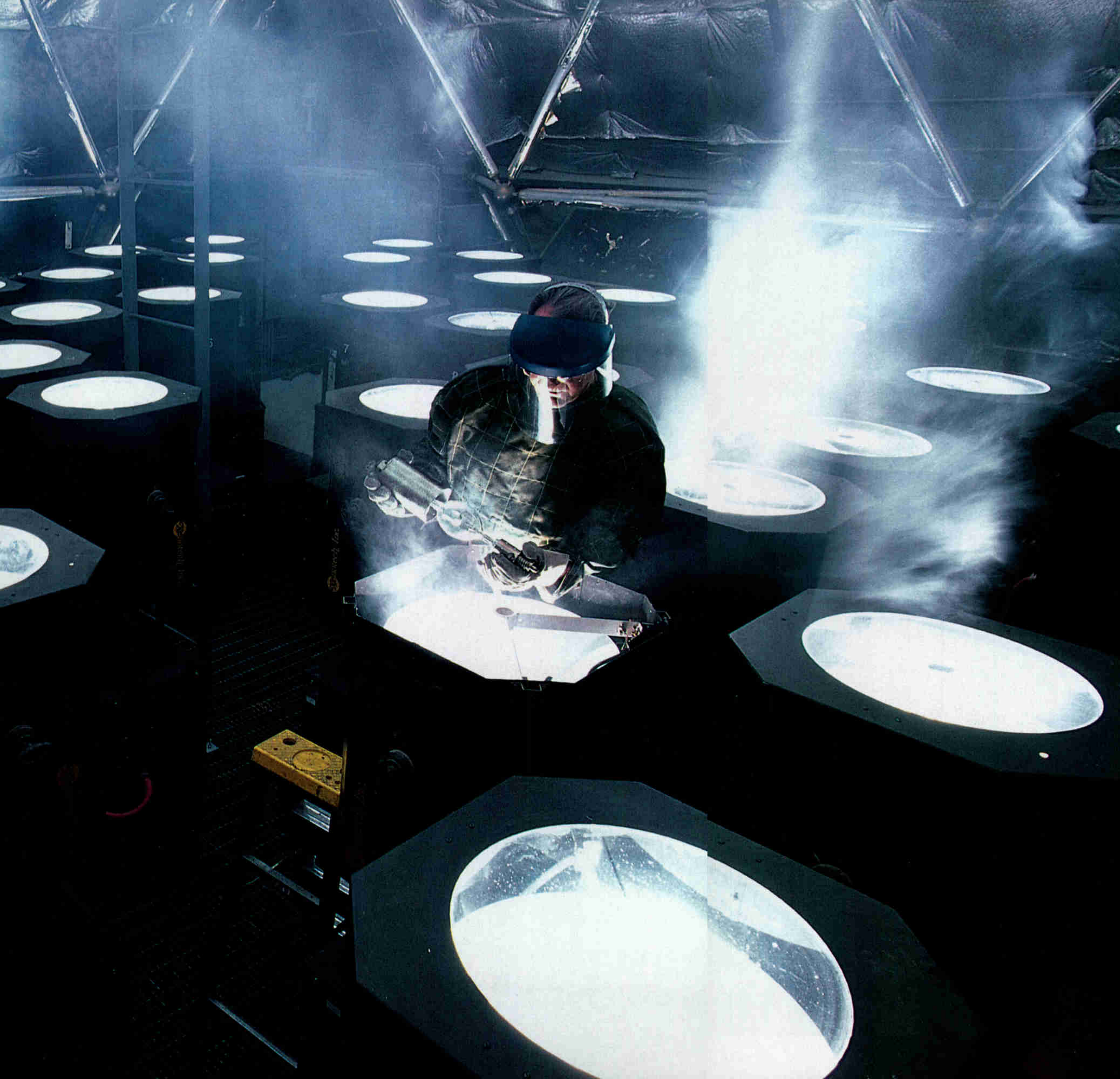
Armored technician Chuck Searcy, Jr., handles one of 39 volatile 7,000-watt xenon lamps atop the Luxor pyramid on the Las Vegas Strip. Touted as the world's brightest light, the Sky Beam is strong enough to read a book by—ten miles out in space. Under high pressure, xenon, a gas, emits a white, sunlike light when an electric current is applied to it. The gaudy radiance of the Strip comes mostly from the gas neon. First used in a light in 1910, neon had revolutionized advertising displays by the mid-20th century.
